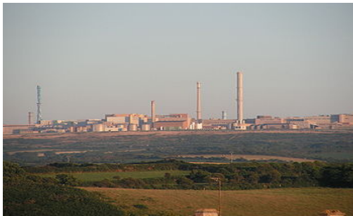
La Hague Reprocessing plant
